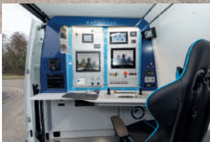
Control room, ProKasro
